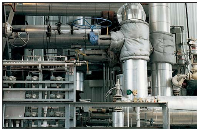
Pressure seal valve in a cogeneration power plant.
